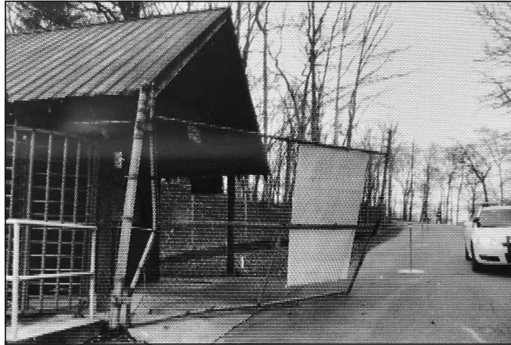
A picture of the damaged front gate at the Georgia Mountain Fairgrounds that somebody drove through over the weekend.
